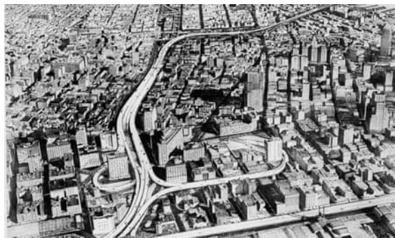
A schematic diagram from 1959 of the proposed Manhattan Expressway, a -10lane highway that required the demolition of 416 buildings. Source: (Reed, 2016).
